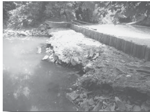
City of Franklin lowhead dam July 2007 - No water flow
