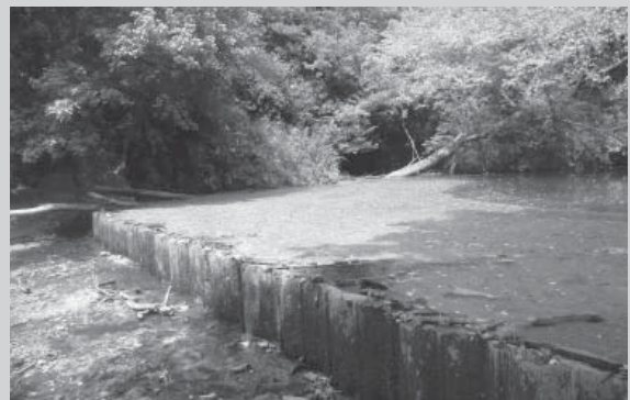
The lowhead dam stops the flow of water during the low-flow summer and fall months.
